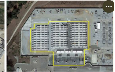
Elkhorn Battery Storage
