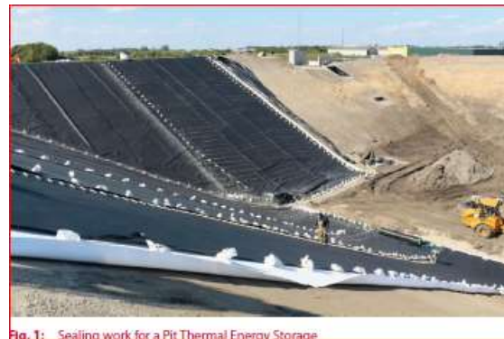
Fig. 1: Sealing work for a Pit Thermal Energy Storage
